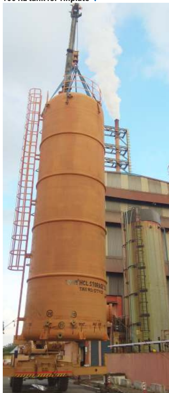
100 KL tank for Tinplate ▼
